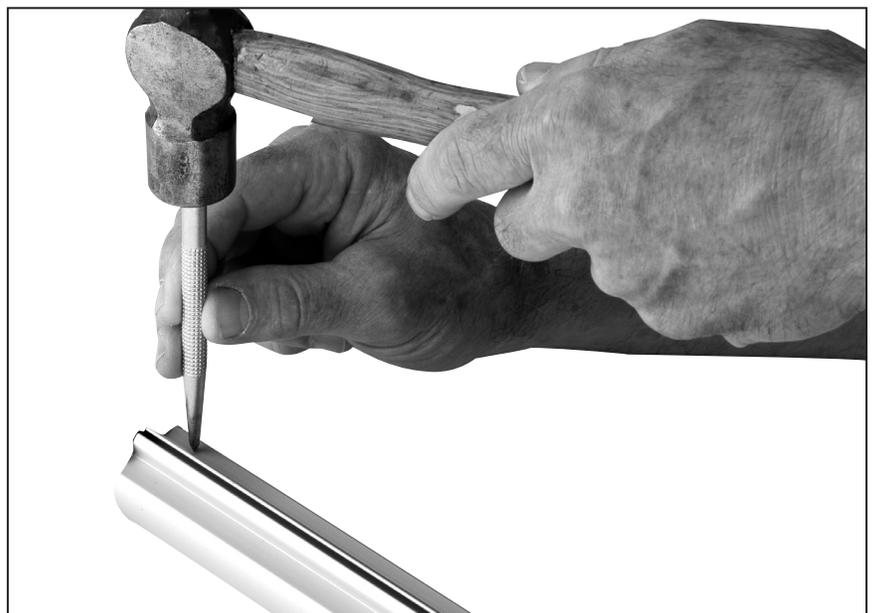
Drill two 1/8" (3 mm) holes in foil for self-tapping screws.
